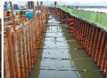
⑤ Tie-Cable 설치
